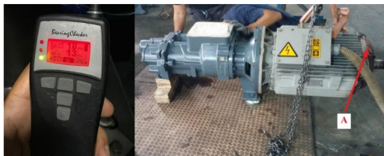
Gambar 6. Pengukuran shock pulse bearing motor A.
